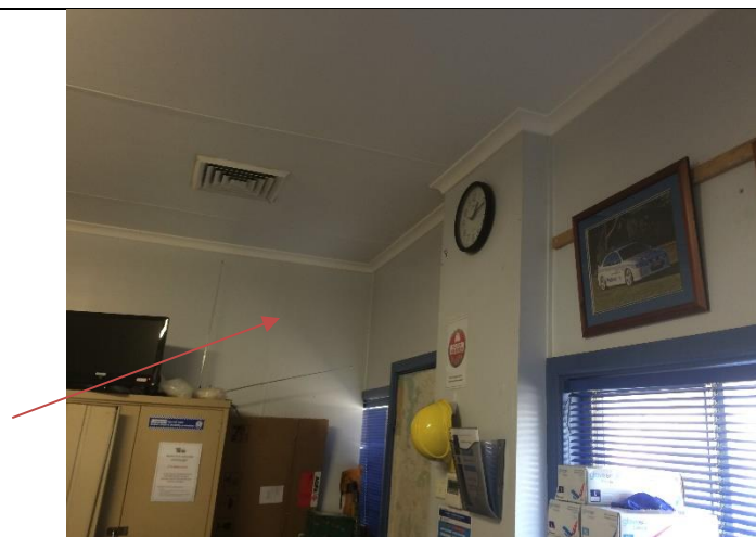
Photo 10: Highway Patrol Office – Internal; Constables Office, walls and ceiling – Asbestos Fibre cement lining (A3)
