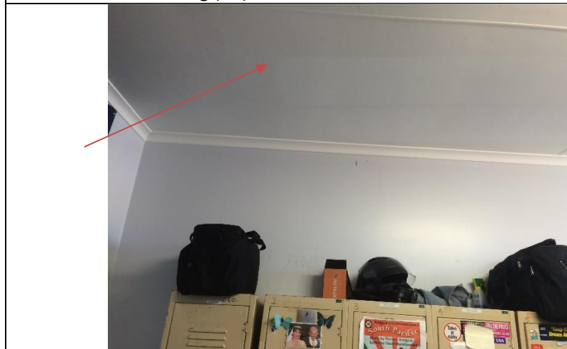
Photo 11: Highway Patrol Office – Internal; Sergeants Office, walls and ceiling – Asbestos Fibre cement lining (A4)
