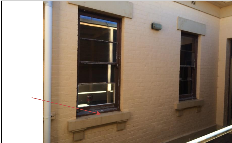
Photo 13: Highway Patrol Office – External; Window frames lower, cream – Lead Paint (A3)
