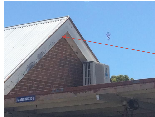
Photo 12: Highway Patrol Office – External; eave, fascia barge boards – Lead Paint (A4)
